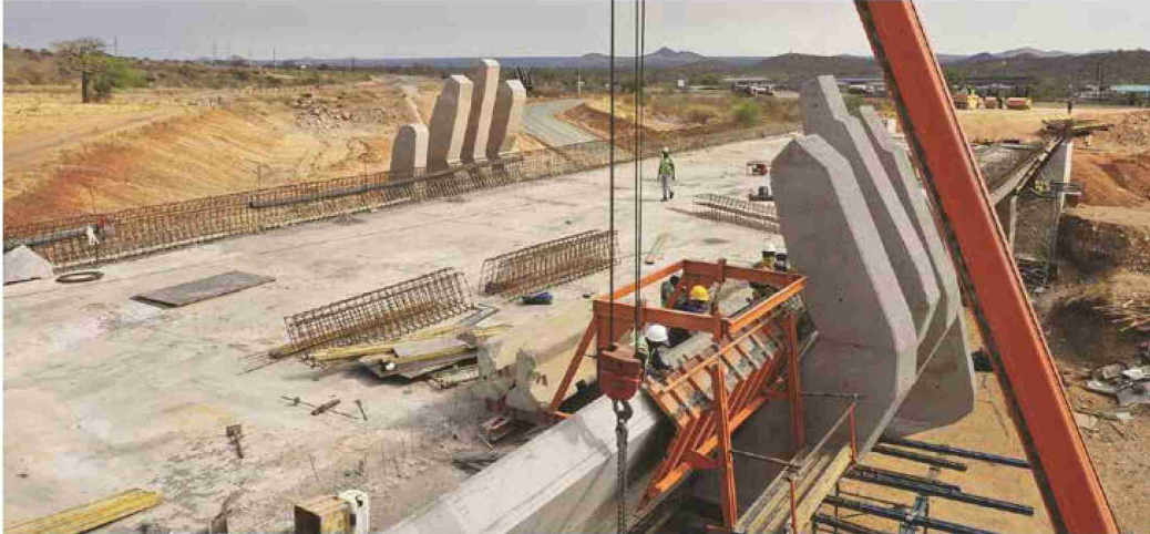
The deck is supported by the columns of the hands.
