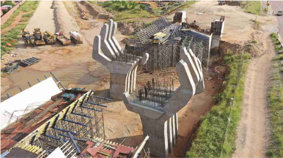
The Nancefield Bridge Project in progress.
