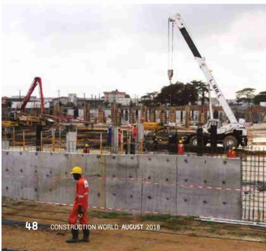
Construction of a retaining wall during phase 1.
