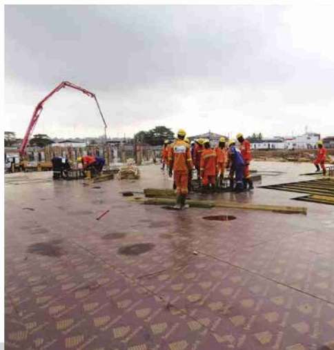
The ground floor slab during phase 1.
