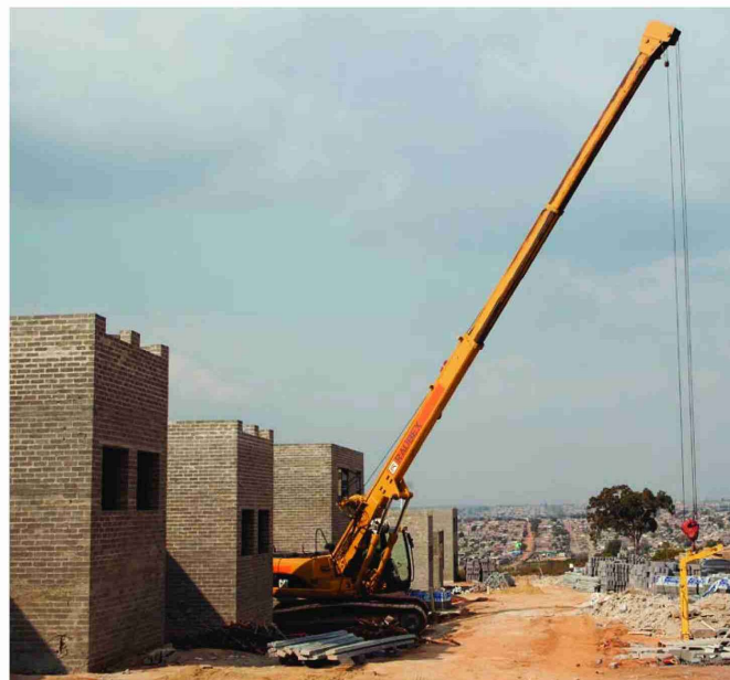
Four-storey RDP units under construction.
