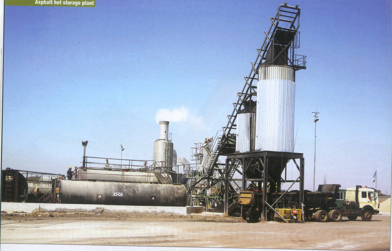
Asphalt hot storage plant
